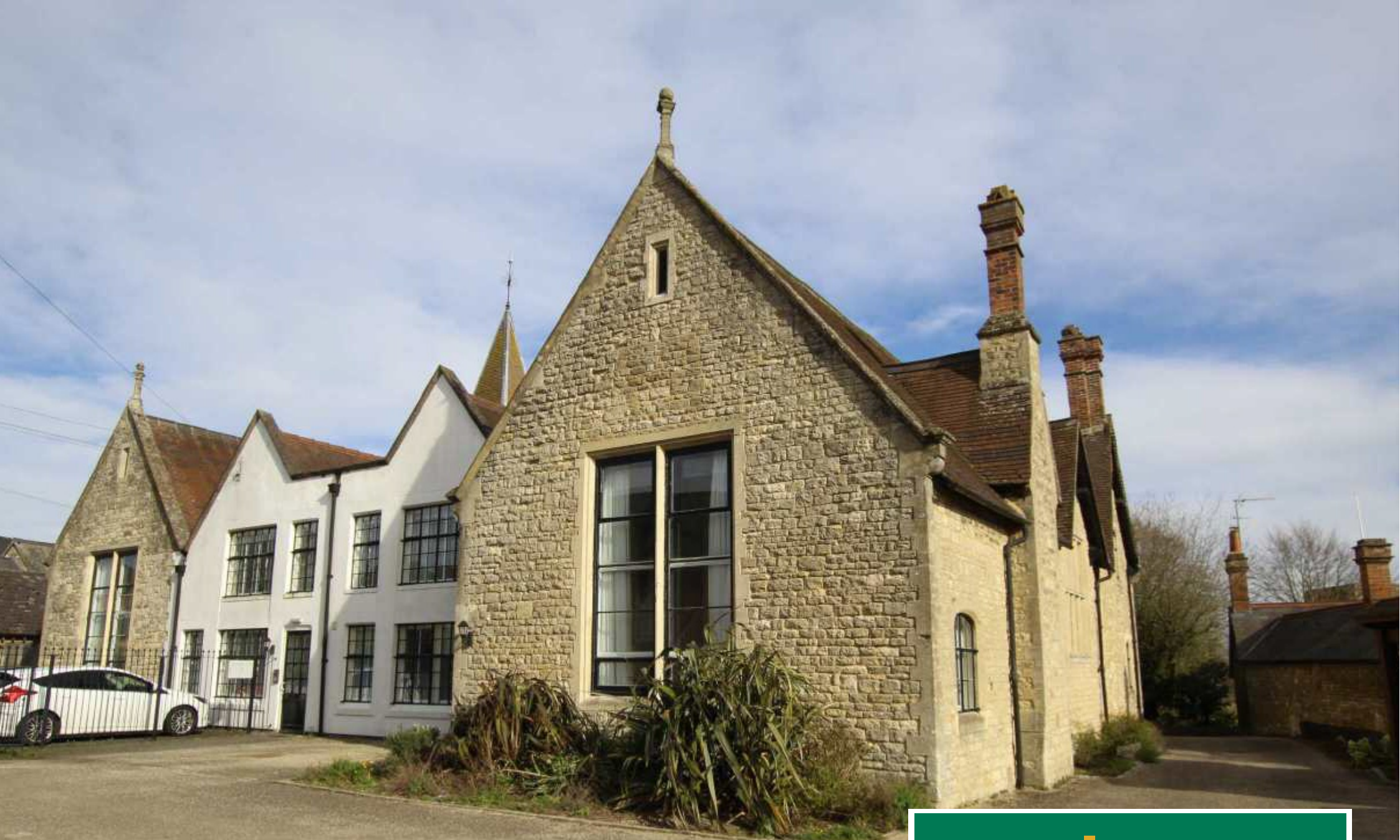
The Bell Tower, Brackley Northants NN13 6AL
